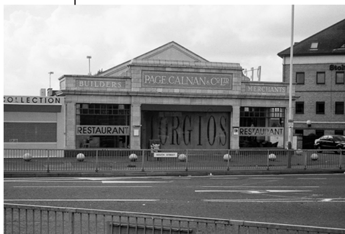
Locally listed Page Calnan building c.1930
