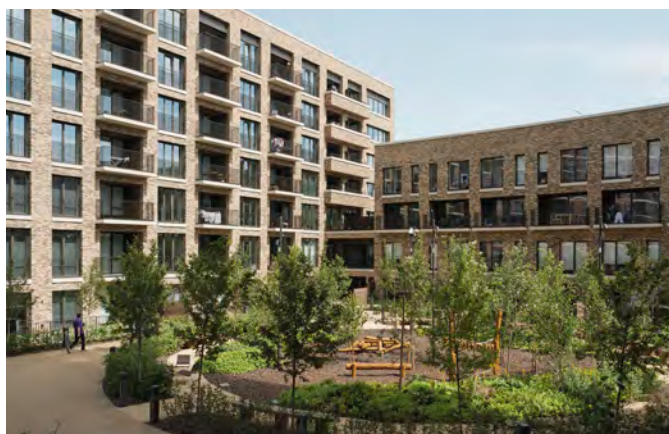
Integrated stacked car parking with communal residential courtyard above – Canada Water, London
