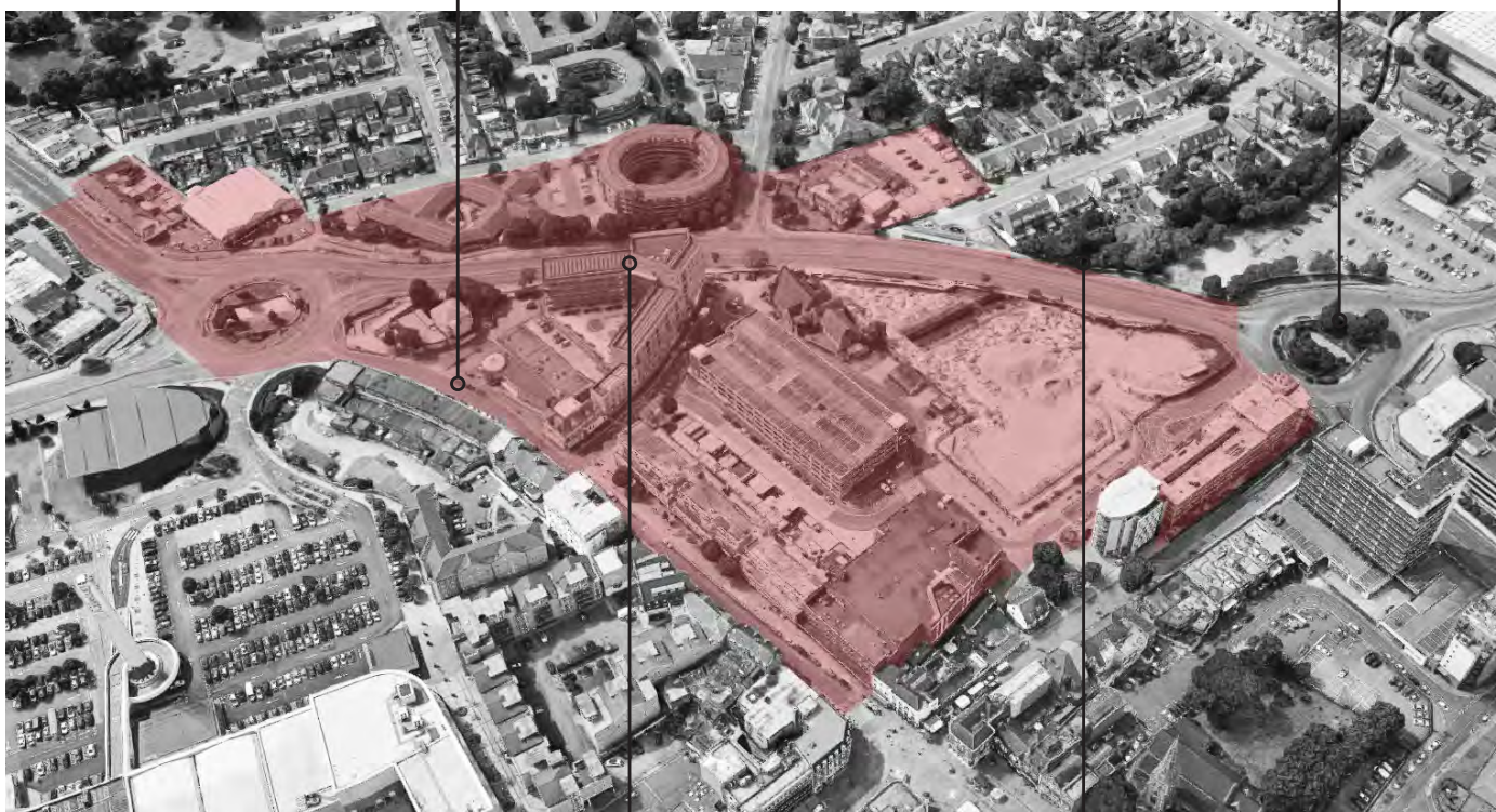
Aerial view - looking North West
