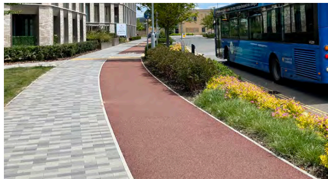
Urban street with space for pedestrians, cyclists, Nature-based SuDS, and public transport – Eddington, Cambridge
