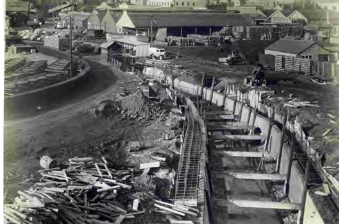
Culverting the River Rom in the Brewery, 1960
