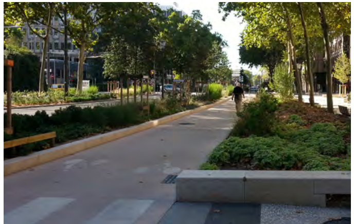
Major street with Nature-based SuDS and segregated cycle lane. Rue Garibaldi, Lyon
