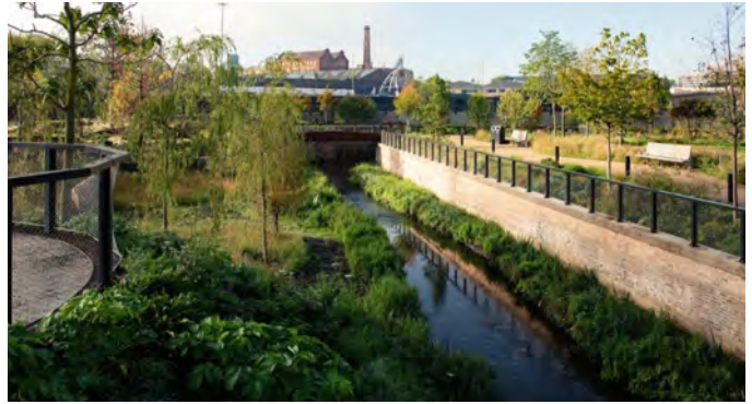
Partially renaturalising the River Rom and creating an active travel link to the town centre – Mayfield Park, Manchester
