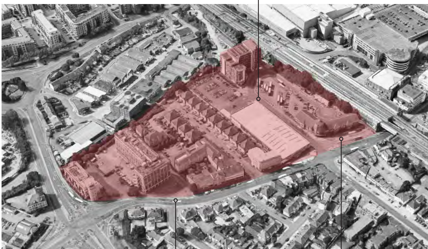
Aerial view - looking North West
