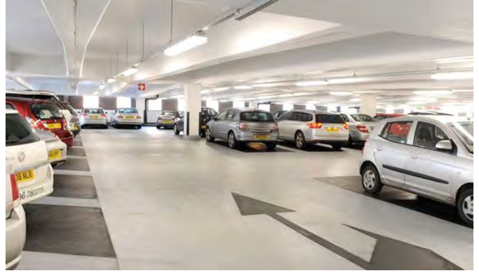
Integrated car parking – High quality, safe car parking in built structures – Q Park, Liverpool
